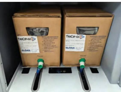
FIGURE 3 Oil container modules.
